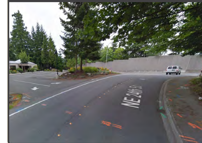
D. NE 24th St at 112th Ave NE, looking east
