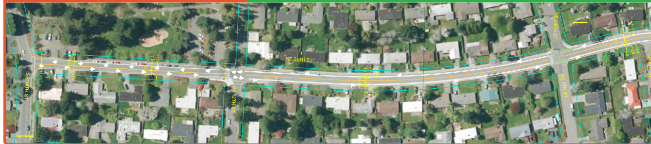
164th Ave SE from SE 14th St to SE 8th St
