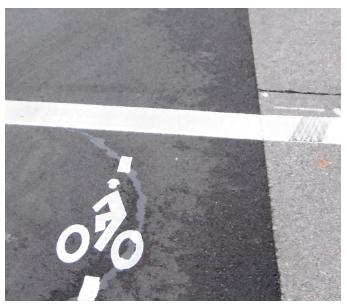
Bicycle Detector Marking at Signalized Intersection
