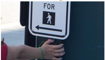
through a green interval if sufficient green time is available in that cycle to allow a pedestrian to cross. The permitted left turn signal phase for vehicles is skipped when a pedestrian is served as an additional safety measure.
