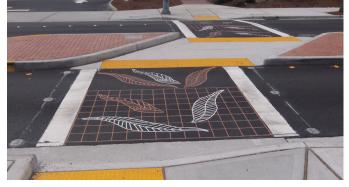
To distinguish the crosswalk from the travel lane and to provide a more interesting and pleasant environment for the pedestrian, special paving is installed in the crosswalk. For added safety the special paving is bracketed by wide and highly visible white lines. The longevity of the pavement design is extended by embedding the decorative pattern into the asphalt so that is it not worn off by vehicle tires
