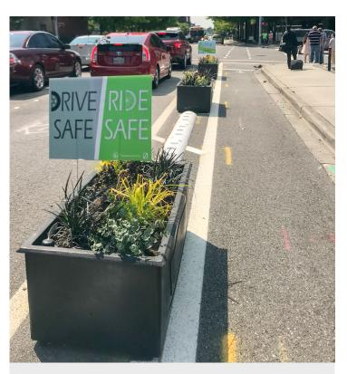
**Figure 5.** Planter boxes were installed in the painted buffer area along several segments of the demonstration bikeway, providing a decorative form of enhanced physical separation.
