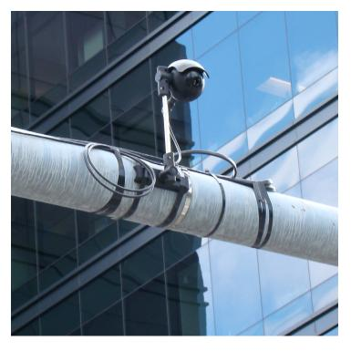
Figure 35. Image of video detection camera
