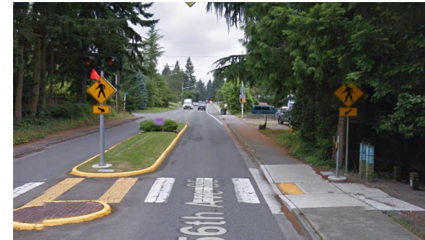
156 th Ave SE, south of SE 27 th St, looking north
