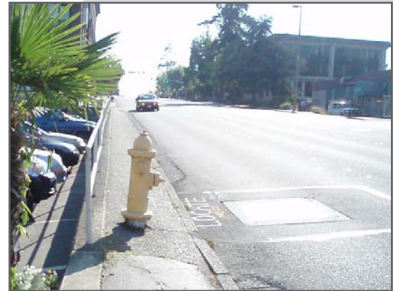
A fire hydrant on this 3 foot sidewalk on the north side of Main Street (between 107th and 106th) renders the entire sidewalk unusable.
