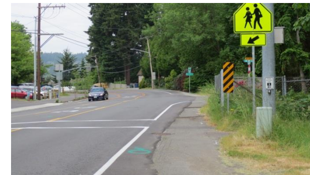
W Lake Sammamish Pkwy, looking north
