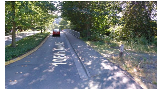
108 th Ave NE and Burlington Northern, looking southwest
