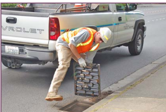
Where bikes may be present, drainage grates what have bars parallel to the roadway are being replaced with a bicycle safe design.
