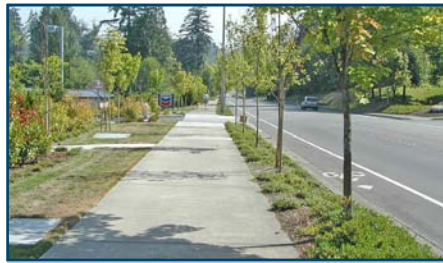
An 8 foot-wide sidewalk and 4 foot-wide planter strip along a Lakemont Boulevard, south of Village Park Drive SE.
