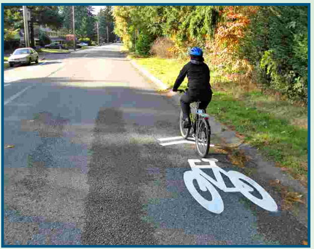
Bellevue's initial "sharrow" experiment on 161st Ave SE is shown to improve both bicycle positioning and motorist behavior.
