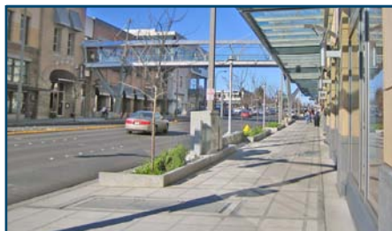
A 12 foot-wide sidewalk and 4 foot-wide planter/furniture strip along 104th Avenue NE, a downtown principal connection.
