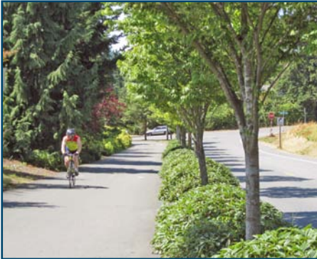
Off-street path running parallel to SE 34th St along the I-90 Trail.
