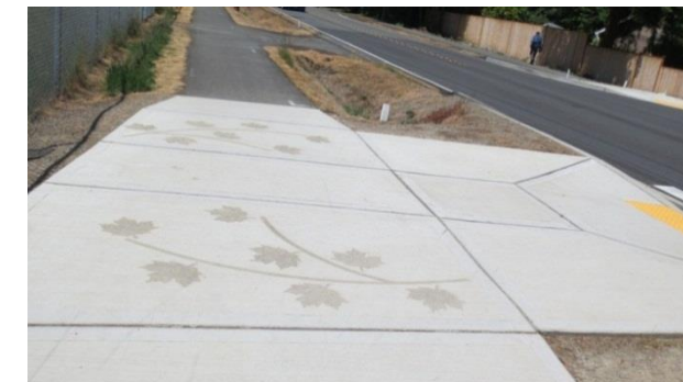
Sidewalk treatment at Northrup Way and 160 th Ave NE
