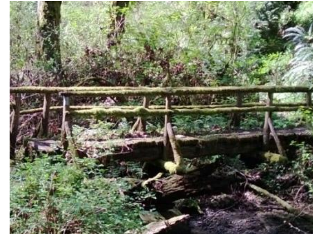
Coal Creek Primrose Loop Trail – 120’ Bridge Phase I
