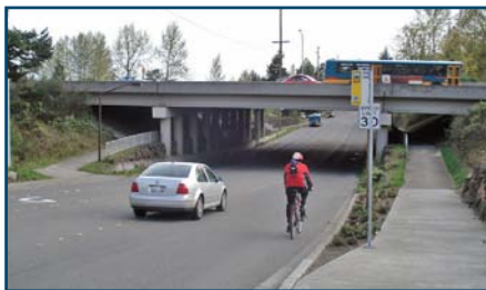
Wide outside lane with no fog line along 116th Ave SE.
