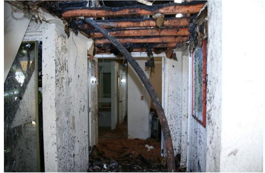
January 26, 2009 12 unit condominium constructed in 1981. Combustible materials too close to a heat source in the attic area, converted to storage space without permits. Damage was estimated to be $160,000
