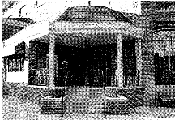
Visual and physical obstructions such as recessed entryway and grade separation
