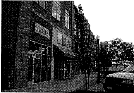
Glazing with simulated divisions that do not connect the sidewalk or street to the interior
