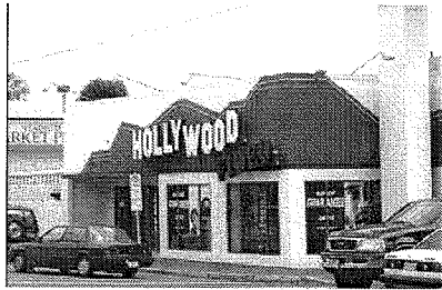
Sign overwhelms the architectural quality of the building
