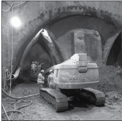
East Link construction begins Page 3
