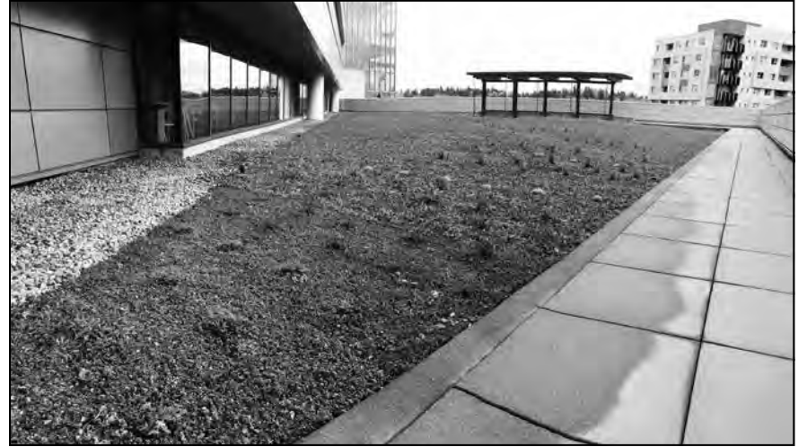
The green roof features drought-tolerant vegetation.
