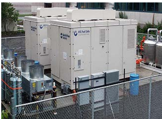
Figure 2-21. Fuel Cell (Soutter, 2012)
