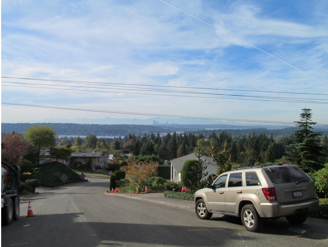
Figure 11-19. 115 kV Existing Overhead Lines in Bellevue Affecting Views of Lake Washington and the Seattle Skyline, from a Distance of 500 feet.
