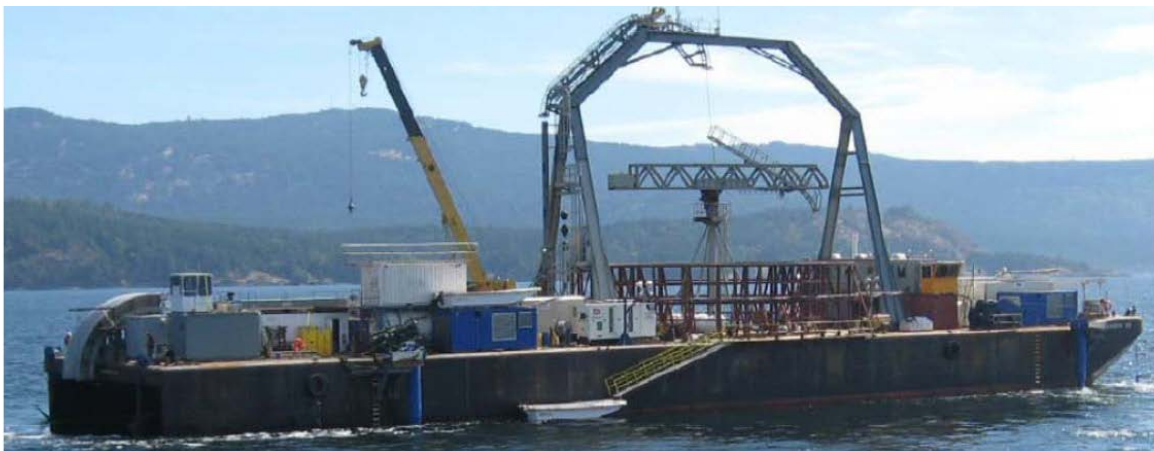
Figure 2-11. Typical Barge for 230 kV Cable Installation (Power Engineers, 2015)
