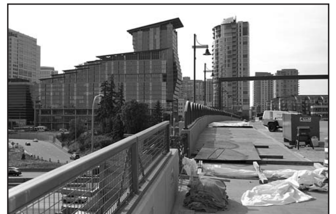
The Northeast 10th Street overpass, near completion.
