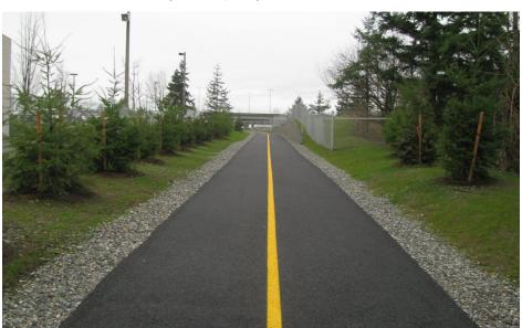
**FIGURE 78** Pervious asphalt on the Pheasant Branch Conservancy trail (Middleton, WI).
