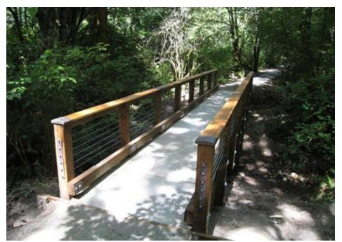
**FIGURE 71** Examples of prefabricated wood and metal bridges with asphalt or concrete decking.
