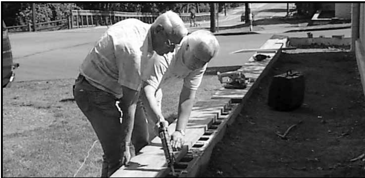
Volunteers work on a retaining wall.
