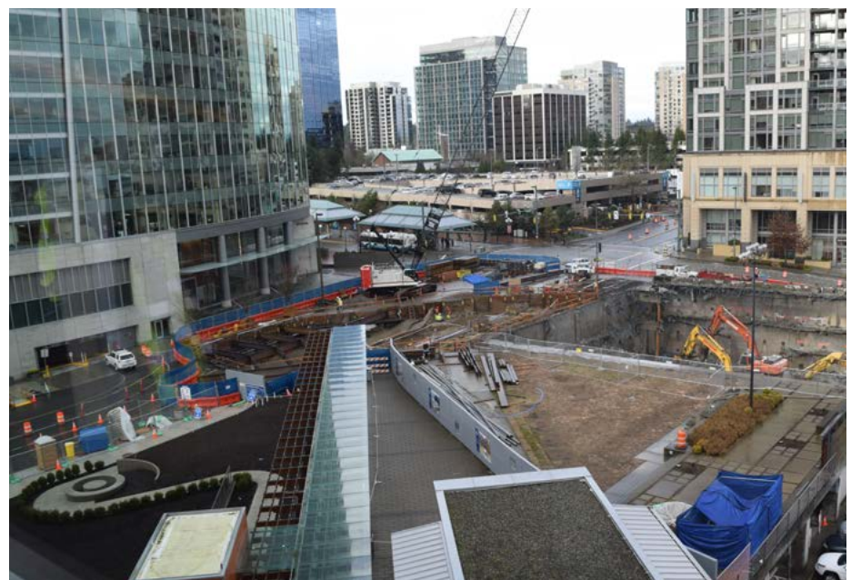
Construction of Bellevue Downtown Station at City Hall.
