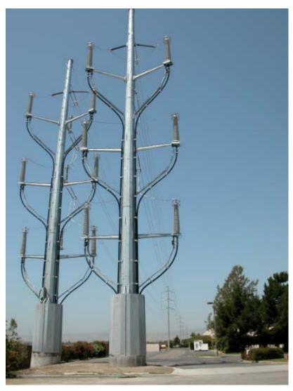
Figure 3-10 Typical 230 kV Riser Structure
