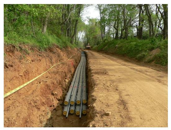
Figure 3-9 Example of duct bank construction in Railroad (retired) Corridor
