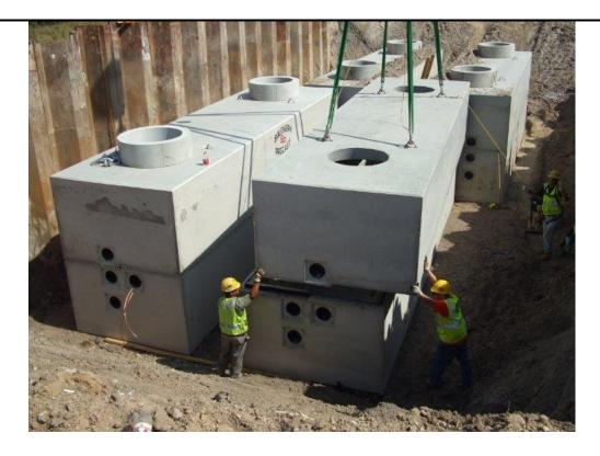
Figure 2-9 Splicing Vault Installation
