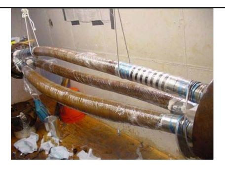
Figure 2-12 Typical HPFF Joint in a Vault
