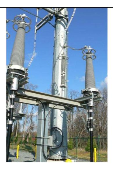
Figure 2-3 Typical 230 kV XLPE Terminations
