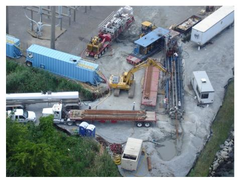
Figure 2-7 Typical HDD Setup
