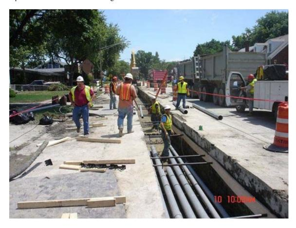
Figure 2-4 Typical trench excavation and duct bank installation (city street)
