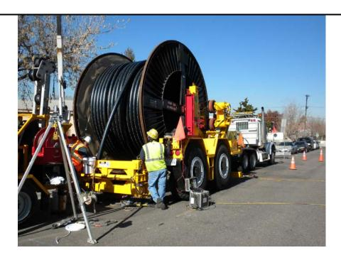
Figure 2-10 Typical Cable Pulling Set up
