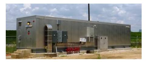
Figure 2-15 Typical Pressurization Plant
