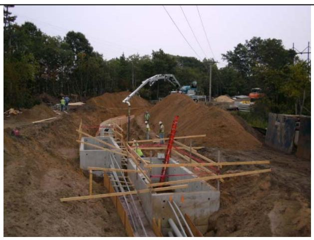
Figure 3-5 Duct Bank and Vault Placement in Rural ROW
