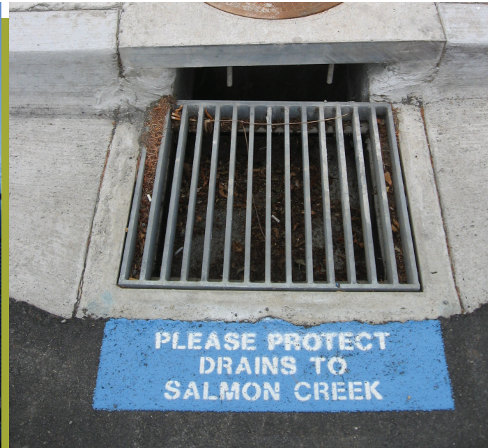
Stormwater inlet
