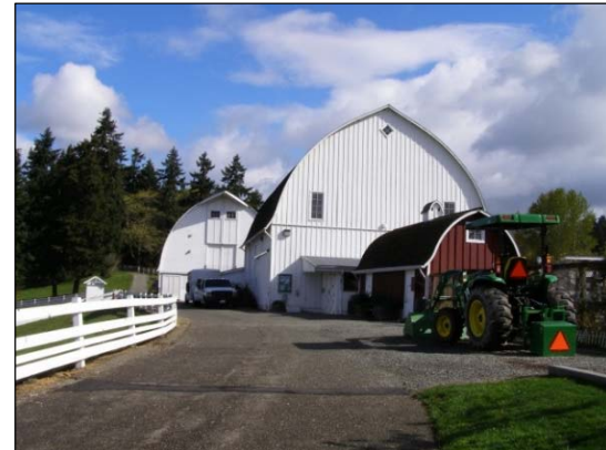
Twin Valley Dairy Barn. Source: DAHP, 2016.
