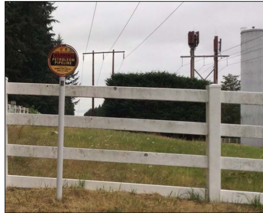
Sign marking location of the Olympic Pipeline in existing corridor (foreground); telecom equipment mounted on existing poles (background)
