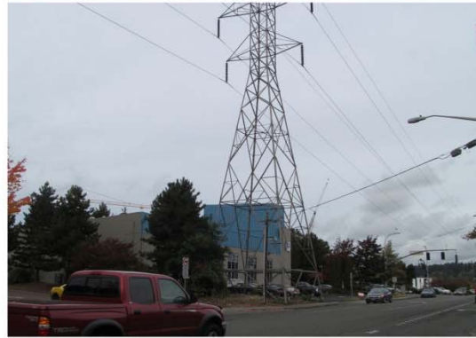
Incompatible height and form with surrounding built environment
