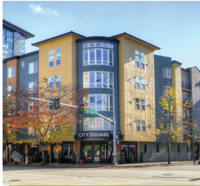
Typical multi-family residential development in Bellevue
