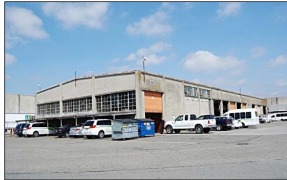
Safeway Distribution Center Truck Repair Building. Source: DAHP, 2016.
