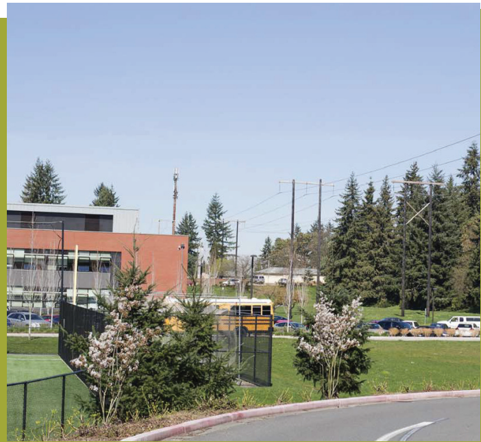
City of Bellevue, existing transmission lines
