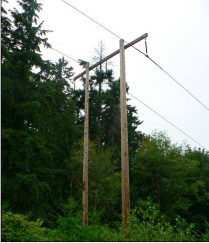
Existing transmission line H-frame structure
