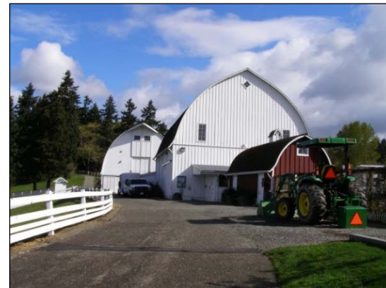
Twin Valley Dairy Barn. Source: DAHP, 2016.
