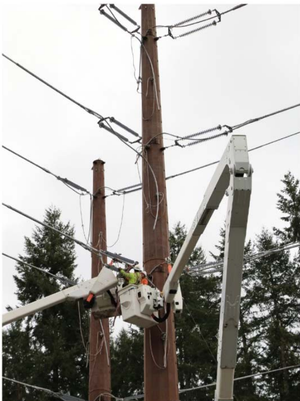
Stringing a transmission line
