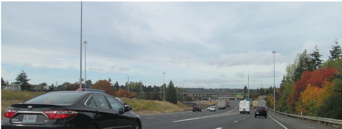
Existing westbound view where Oak options would cross I-90
