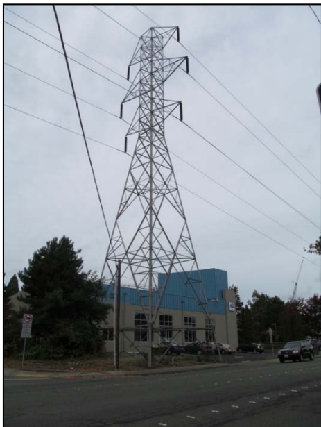
230 kV steel lattice tower in the study area, owned and operated by SCL
