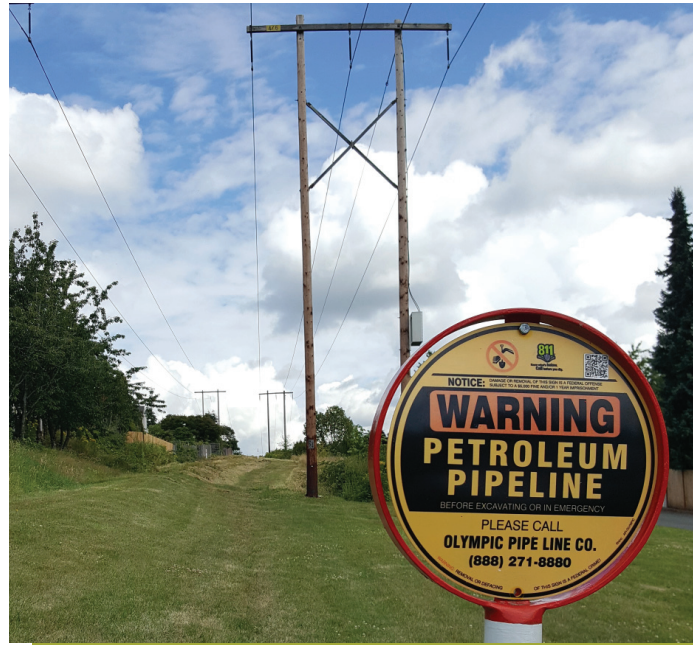
Pipeline warning sign in the existing corridor
