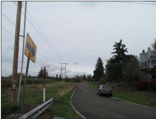
Existing transmission line, looking north on 136 th Ave NE
