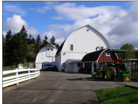
Twin Valley Dairy Barn. Source: DAHP, 2016.
