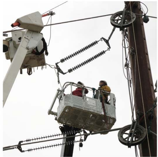
Workers connecting a transmission line to insulators
