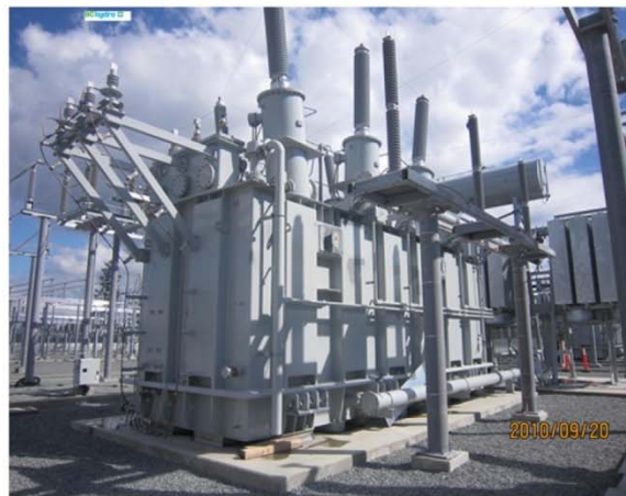
230 kV Transformer
