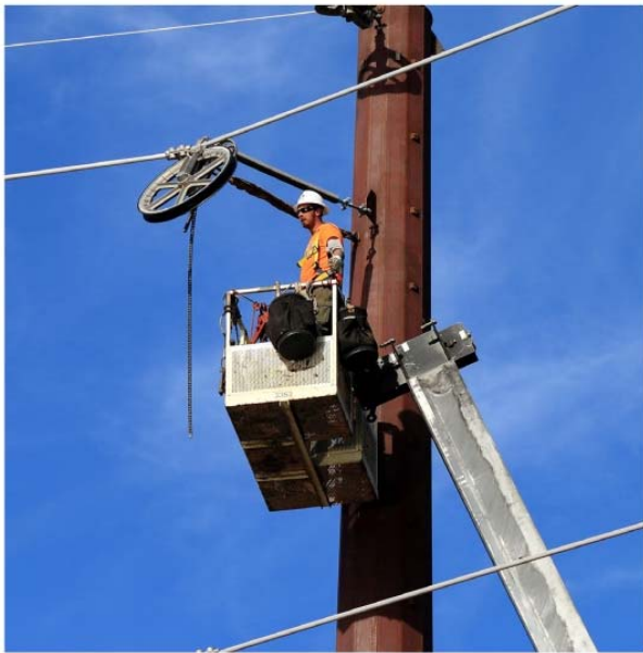
Worker rebuilding a transmission line
