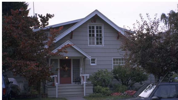
Figure 12 Retrofit using the prescriptive requirements for a remodeled two-story home (attic remodeled, dormers and occupied floor added) provided pony wall less than 18 ½ inches. (Photo by Linda Noson, AGRA Earth & Environmental)
