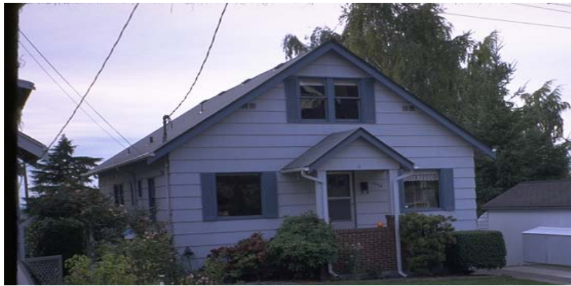
Figure 11 Retrofit using the prescriptive requirements for a two-story home (attic remodeled for occupancy) provided pony wall less than 18 ½ inches. (Photo by Linda Noson, AGRA Earth & Environmental)
