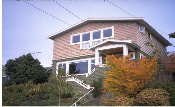
Figure 13 Retrofit using the prescriptive requirements for a three-story home (two-stories plus pony wall over 18 ½ inches). (Photo by Linda Noson, AGRA Earth & Environmental)
