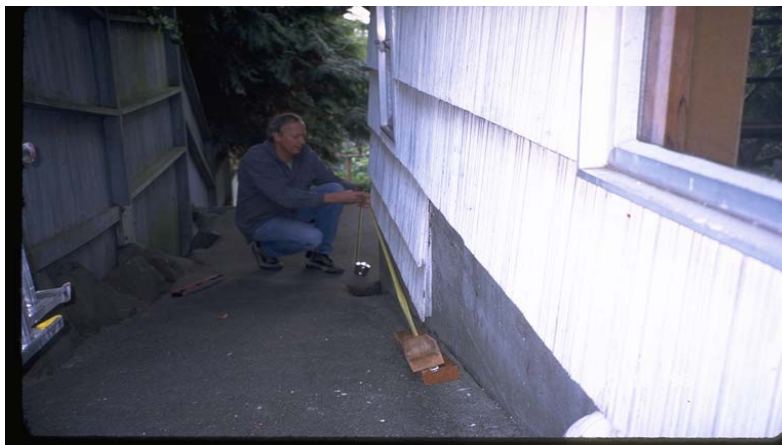
Figure 5 Measuring the horizontal and vertical distance to determine if the home qualifies to use the Standard Earthquake Home Retrofit (SEHR) Plan. This home qualifies to use the standard plan. (Photo by Linda Noson, AGRA Earth & Environmental)
