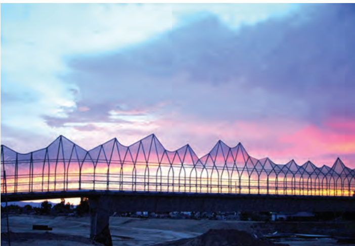
Laurie Lundquist, Mountain Pass Pedestrian Bridge , Phoenix, AZ
