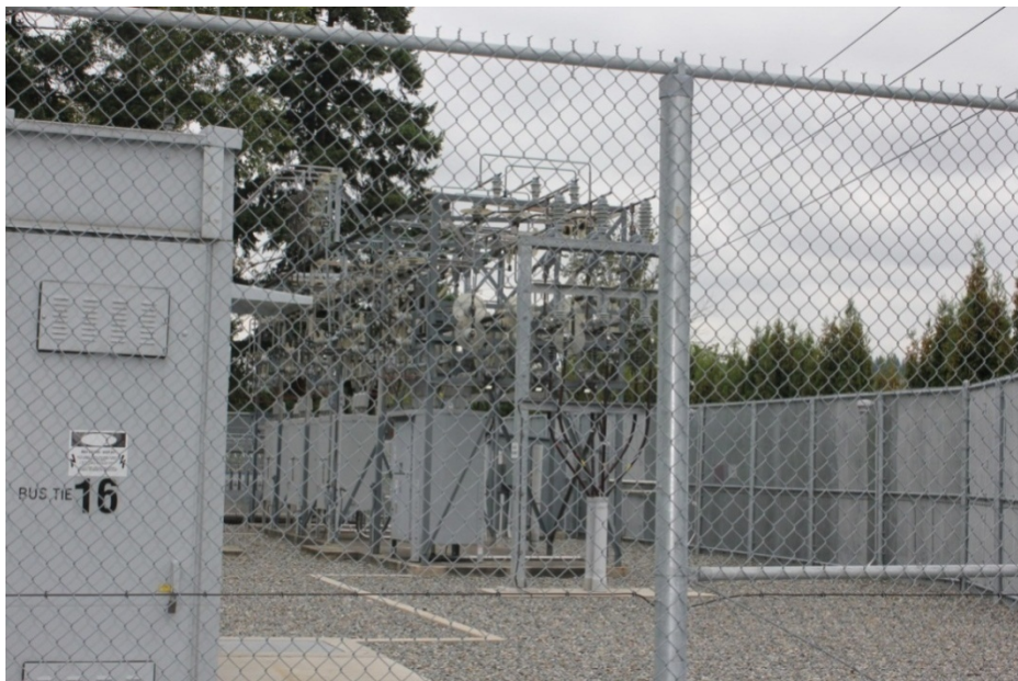
Figure 45. 15 kV Open Air & Metal Clad Switchgear in Factoria Substation
